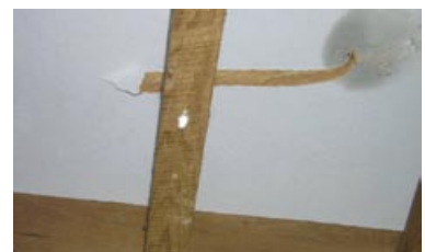
Figure 25 Chrysotile paper on strawboard ceiling panels
