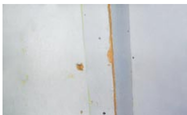
Figure 24 Chrysotile paper on fibreboard boxing
