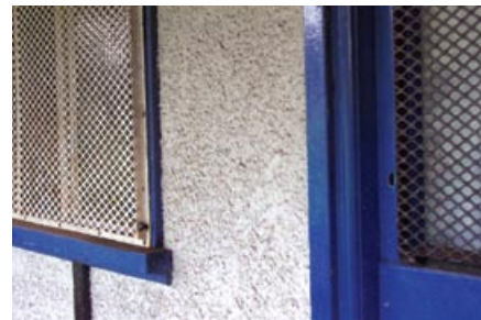
Figure 33 Chrysotile pebble-dash exterior wall coating
