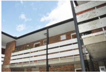
Figure 18 AIB exterior panel on open walkway
