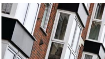
Figure 16 AIB exterior painted panel
