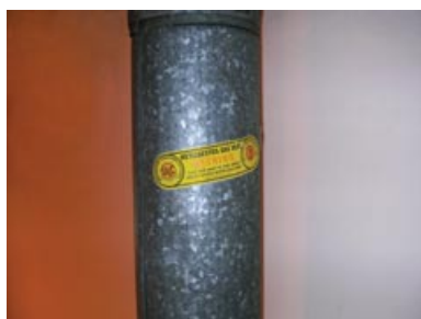
Figure 43 Metal clad gas flue containing chrysotile lining
