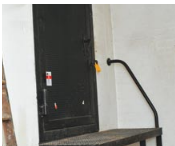
Figure 45 'Durasteel' composite steel and asbestos fire door
