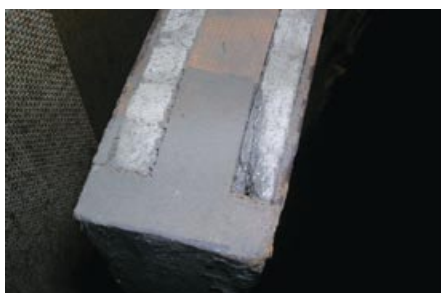
Figure 14 Asbestos panels inside fire door
