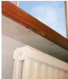
Figure 20 AIB panel between radiator and window
