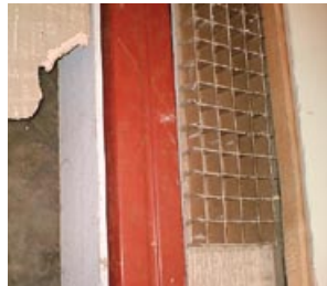
Figure 21 AIB column fire protection in CLASP building
