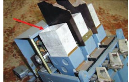
Figure 49 Electrical switchgear with asbestos flash protection
