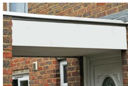
Figure 15 AIB panel in porch
