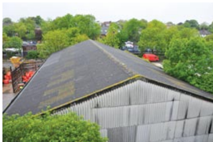
Figure 32 Asbestos cement roof and cladding
