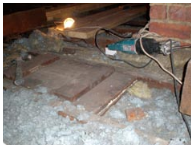
Figure 6 Loose asbestos used as loft insulation
