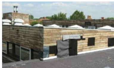
Figure 23 AIB fascia panels with wood effect finish
