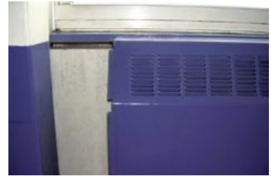
Figure 19 AIB behind school radiator unit
