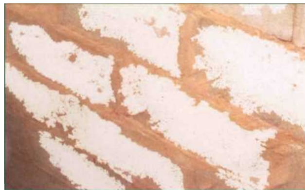
Figure 6.5 Remnants of asbestos on breeze blocks
