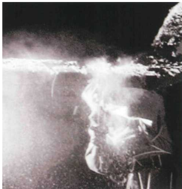
Figure 7.1 Uncontrolled dry stripping
