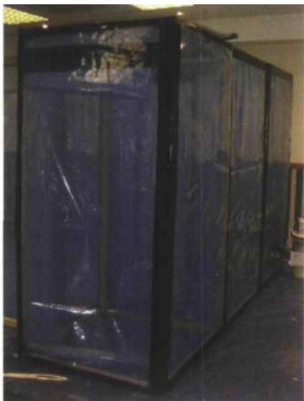
Figure 6.12 Flap arrangements for airlocks
