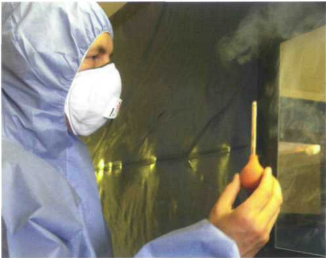
Figure 2.3 Supervisory licence holder checking the integrity of an enclosure
