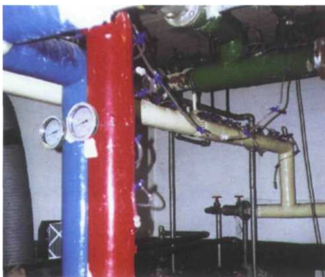
Figure 7.9 Good practice: Wet injection on pipework
