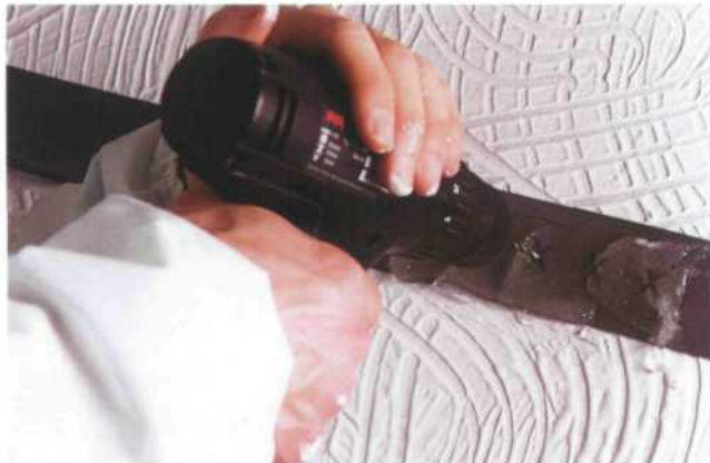
Figure 7.7 Textured coating being drilled through paste
