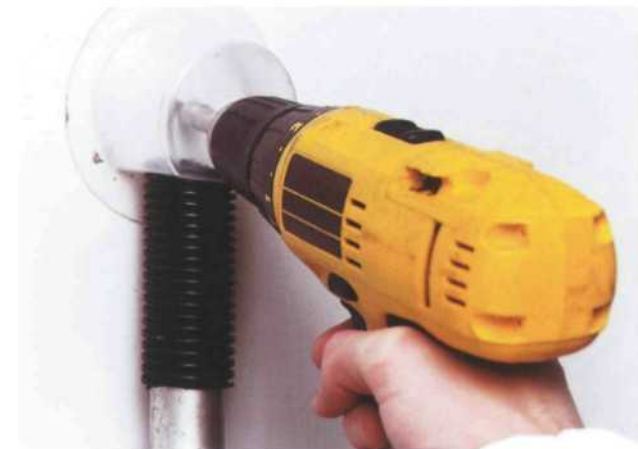
Figure 7.6 Drilling using a low-speed drill with cowl and fitted with LEV
