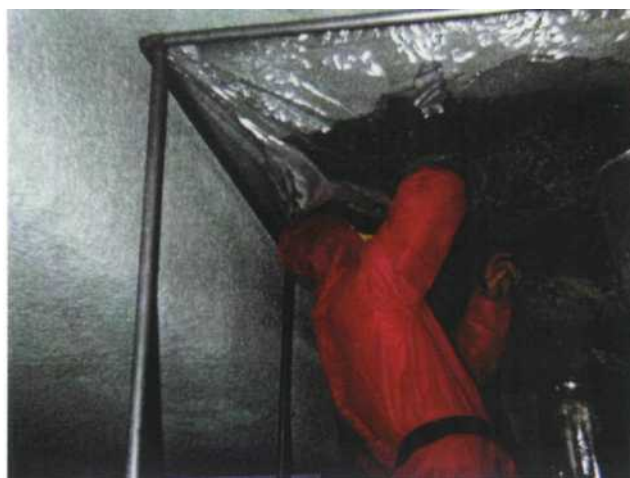
Figure 7.17 A sprayed asbestos coating being removed using a specialised glovebag within a traditional enclosure (the dark area is where the asbestos has been removed)
