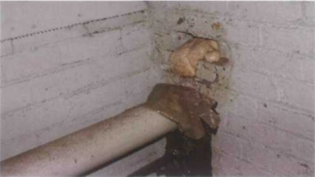
Figure 6.4 An enclosure sealed with expanding foam
