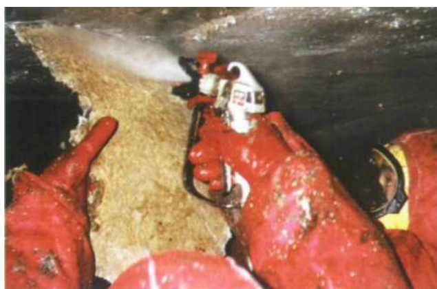
Figure 7.15 Spraying thin coating
