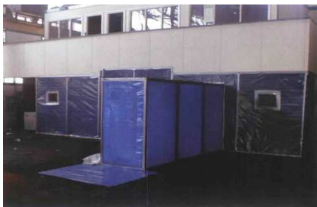
Figure 6.1 Enclosure with three-stage airlock
