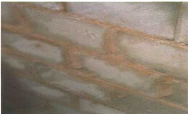
Figure 7.26 Remnants of asbestos on breeze blocks
