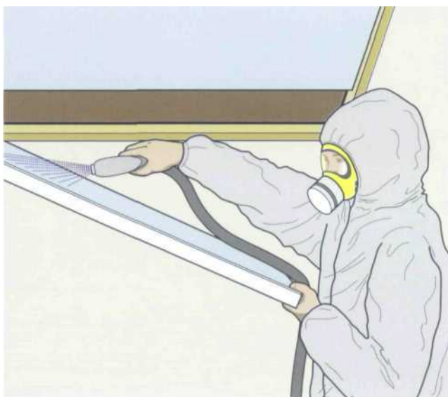
Figure 7.13 Spraying AIB
