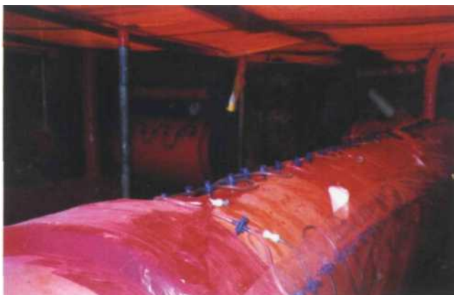
Figure 7.9 Good practice: Wet injection on pipework
