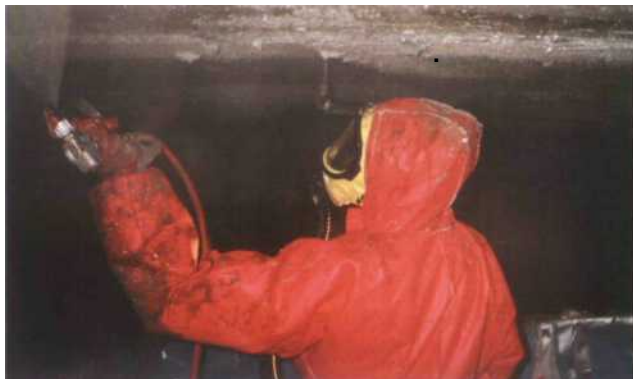
Figure 1.6 Controlled removal of asbestos
