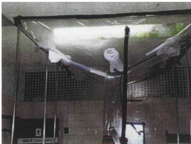
Figure 7.18 A glovebag designed for the removal of sprayed asbestos coatings. Note the gloveports, waste chute and vacuum nozzle used for cleaning and providing slight negative pressure
