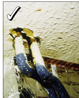
Damaged textured coating, asbestos cement roofing and an asbestos-containing gasket
